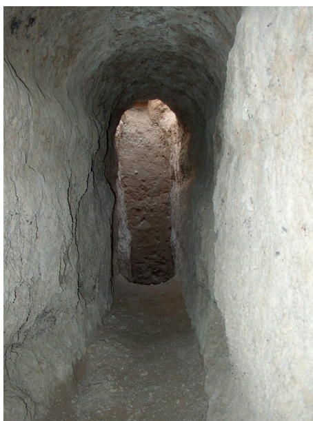
Fig. 15: Under-ground water channel “Falaj” at Thuqeibah.
